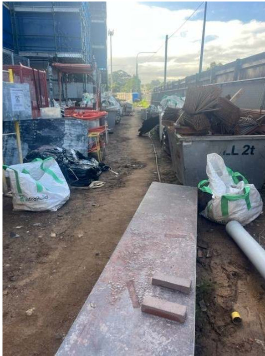
Photos 6&7: Material storage inside the site boundary – ERSED controls in place along the fence line with low risk of sediment escape from site
