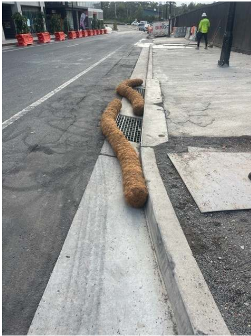
Photo 1: Conferta Avenue clean with no signs of tracking and drain protection in place
